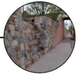
Ca. 1935: Masonry drainage feature and culverts (HR12-14)
