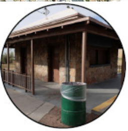
Ca. 1935: Concession Building (HR17)
