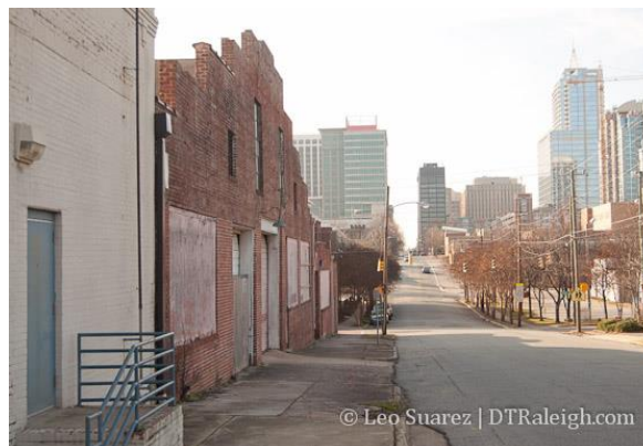
Before: Stone Warehouse, 2014
