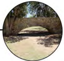
1922: Masonry Arch Footbridge (HR1)
