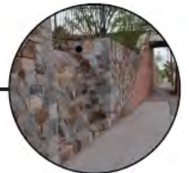
Ca. 1935: Masonry drainage feature and culverts (HR12-14)
