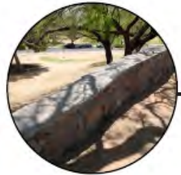
Ca. 1935: Hilltop Garden masonry walls (HR3)
