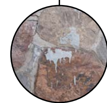
applied paint (masonry)
