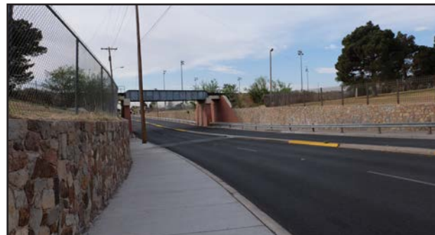
Masonry walls at North Copia Street
