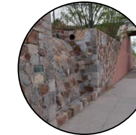
Ca. 1935: Masonry drainage feature and culverts (HR12-14)
