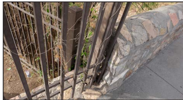
Curved top at the masonry walls
