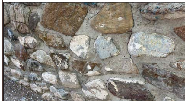
Typical mortar and masonry
