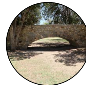
1922: Masonry Arch Footbridge (HR1)
