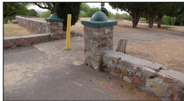
Typical mortar and masonry
