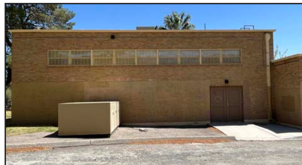
Rear of Garden Center
