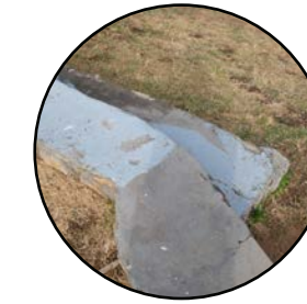
non-historic paint coatings
