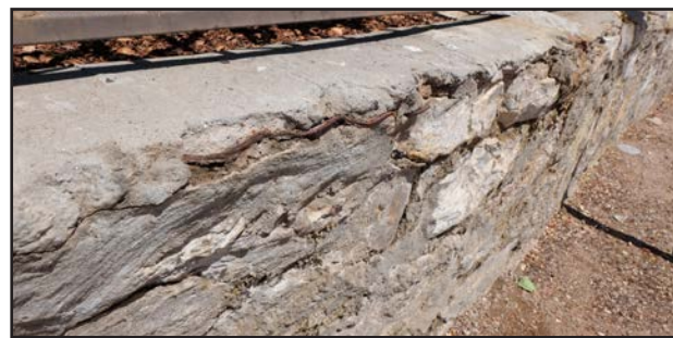
Typical mortar and masonry
