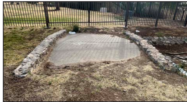
Top of culvert bridge
