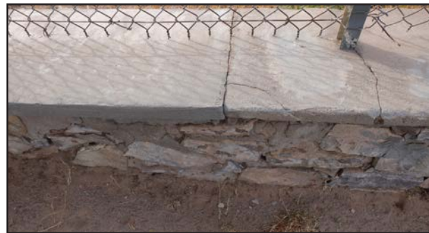
Typical mortar and masonry
