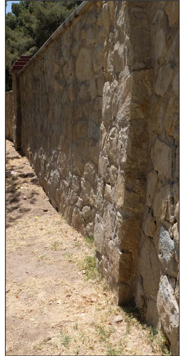
Masonry Walls at the Estrella Street Bridge
