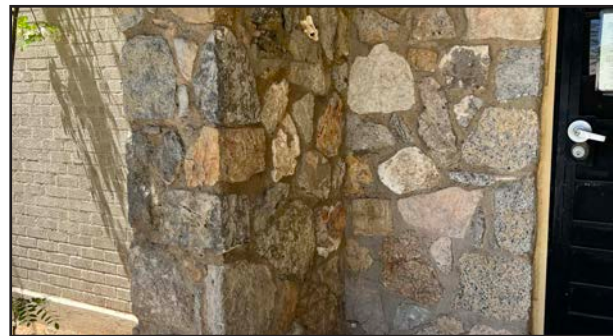
Masonry wall at Garden Center entrance
