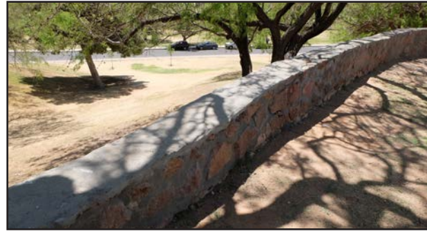
Masonry walls follow the topography of the landscape.
