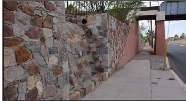
Drainage feature at North Copia Street and the railroad tracks
