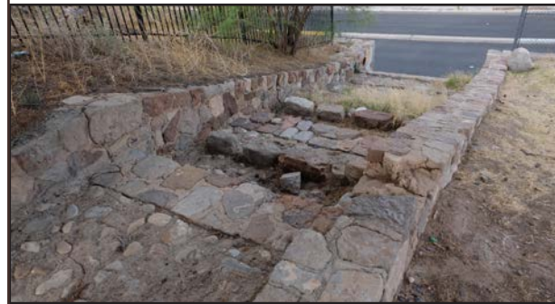
Canal above the drainage feature
