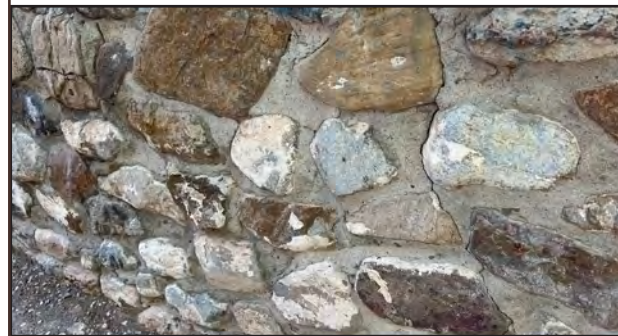
Typical mortar and masonry
