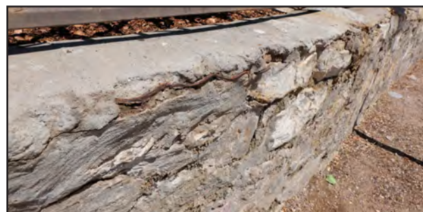
Typical mortar and masonry
