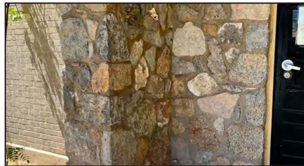
Masonry wall at Garden Center entrance
