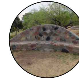
Ca. 1935: Masonry walls, staircases, entrance gates, and benches (HR4-14)
