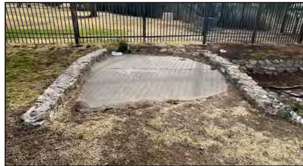
Top of culvert bridge
