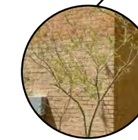
non-historic paint (brick)
