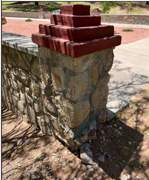
Tiered posts at Estrella Street Bridge
