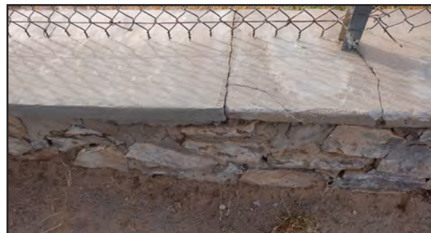
Typical mortar and masonry
