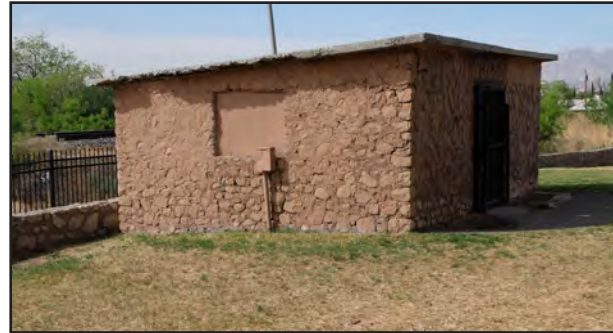
Accessory building exterior with enclosed window
