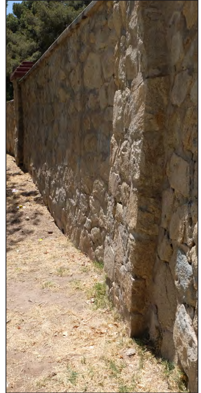
Masonry Walls at the Estrella Street Bridge
