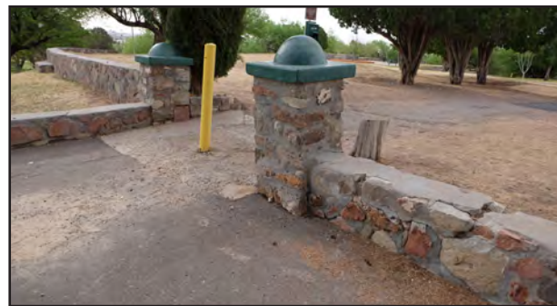
Typical mortar and masonry
